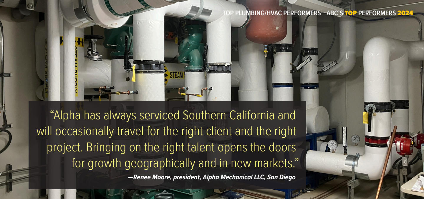
Alpha Mechanical LLC's steam heat exchanger portion of a total HVAC system on the Department of Veterans Affairs' Long Beach Community Living Center.
