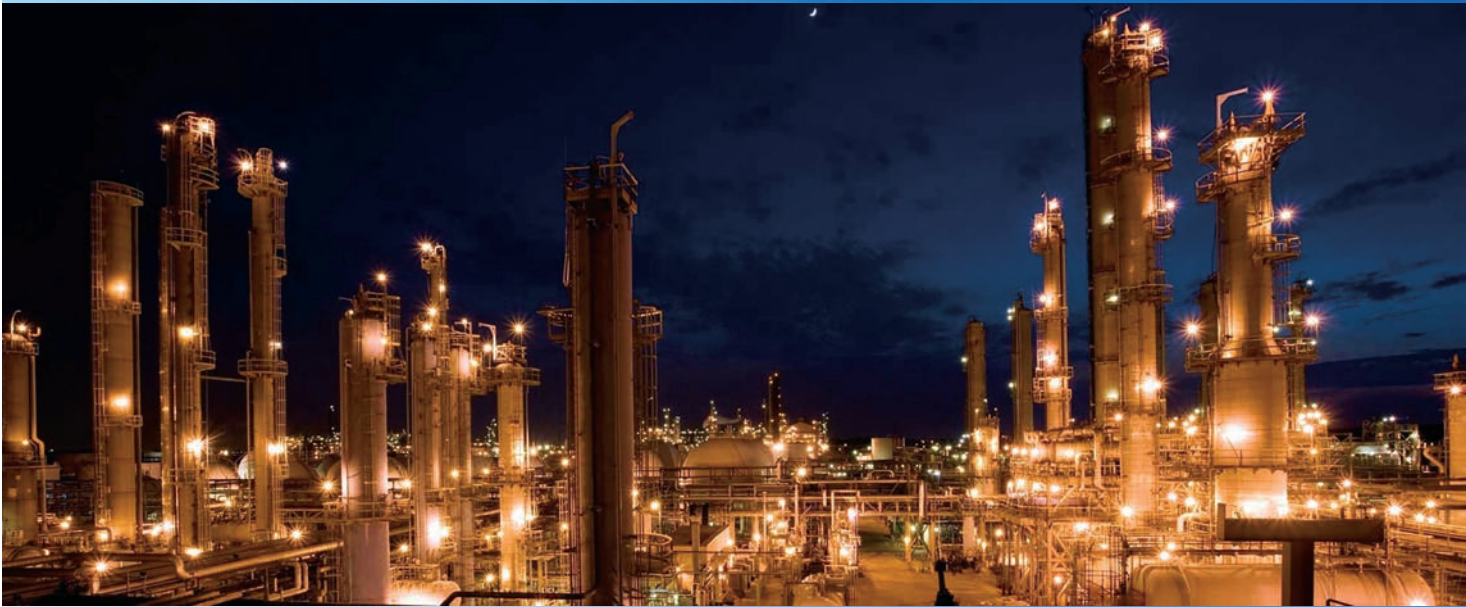
LyondellBasell PO/TBA Project, Apache Industrial, Houston, Texas, ABC National Excellence in Construction® Award Winner
